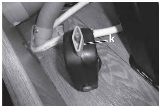
Safety valve for boiler (Frost Control)
